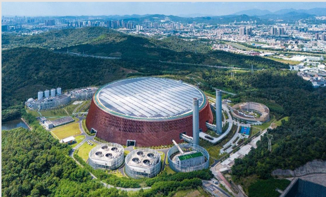
Fig. 11 Longgang Eco-Energy Park
