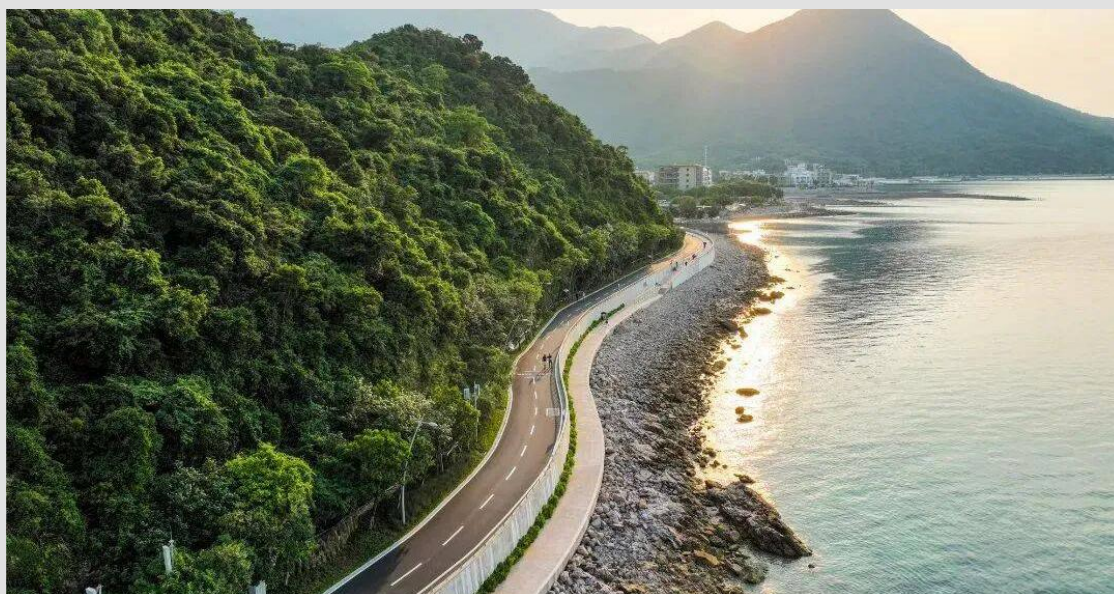
Fig. 12 Yangmeikeng Section of the Phase III Reconstruction Project of Eastern Seawall
